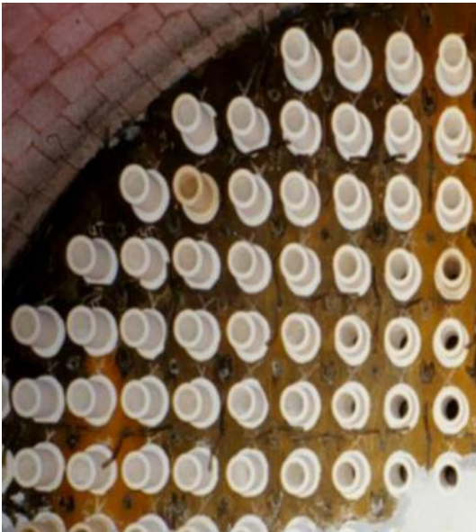
Conventional Ferrules before Final Refractory Installation
